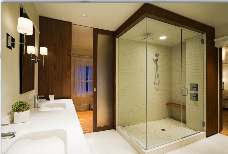
Wall-Mount Hinge System, Recessed Channel-Set Panels
