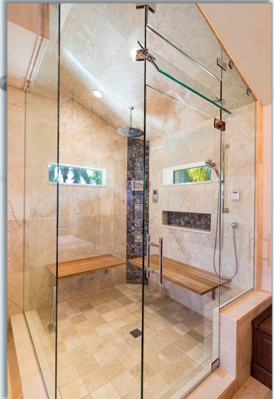
Pivot Hinge System, Clip- and Channel-Set Panels
